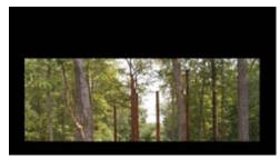
The six tree-like poles support the roof with tension cables, literally tying the structure to its site. Materials were found locally, including the poles that were installed by the local county utility company. To create the 25-foot clear span without the cost of gluelaminated beams, standard
