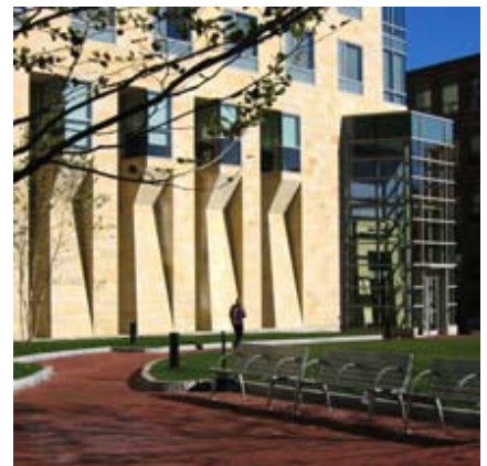
Stull and Lee, John D. O'Bryant African-American Institute at Northeastern University, photo courtesy of architect
