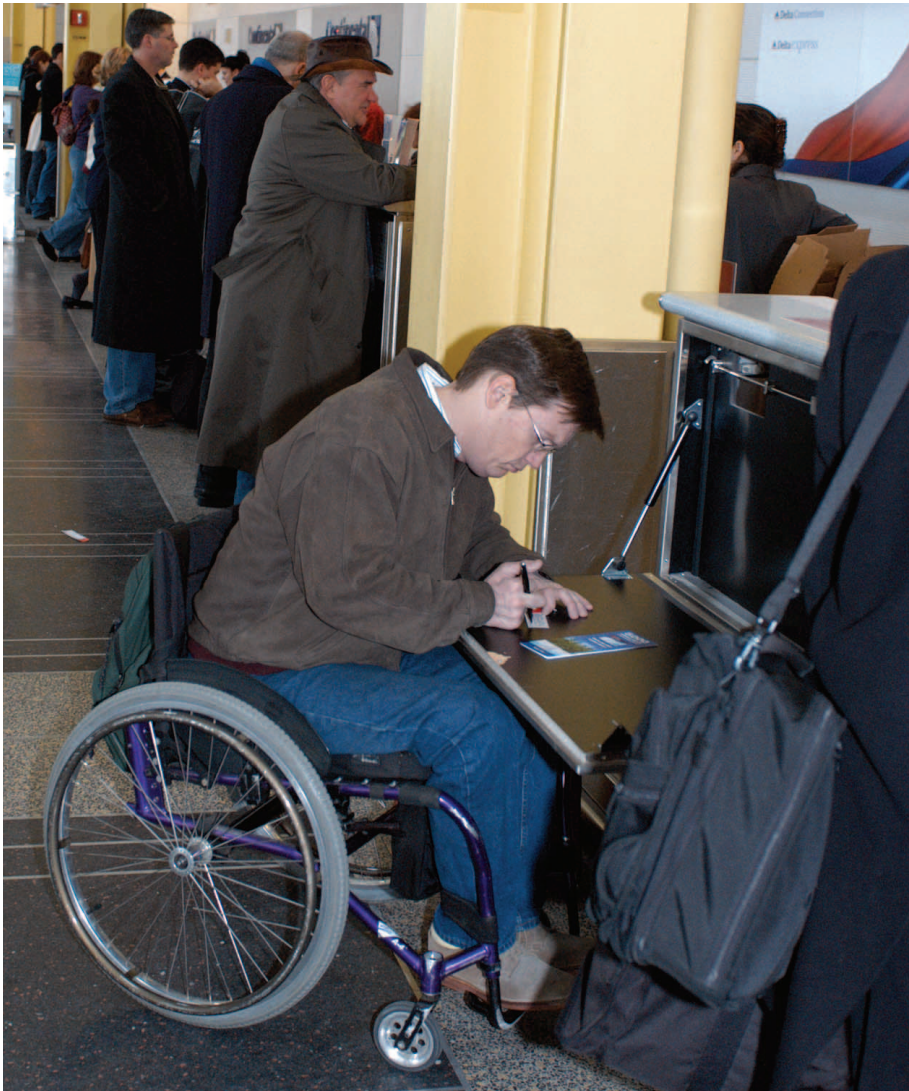
Ticket counters have flip-open panels, providing a lowered writing surface for wheelers.
