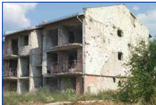
Rough concrete frames are all that remain of most homes in Bosnia, the author reports.
