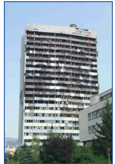
A building in shambles, an all too familiar sight in Bosnia-Herzegovina.
