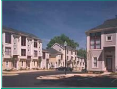
Park West employs varied massing to break up the bulk of 30 units on a 1.8-acre site. Photo © Tim Buchman.
