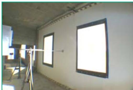
DrChecks helps the State Dept. upgrade security at overseas embassies. Protective measures include special blast-resistant wall and window treatments.
