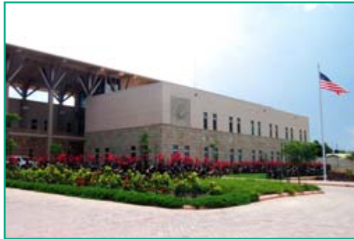
DrChecks had a payback of less than a year on one State Department project. Images courtesy of the U.S. Army Corps of Engineers.
