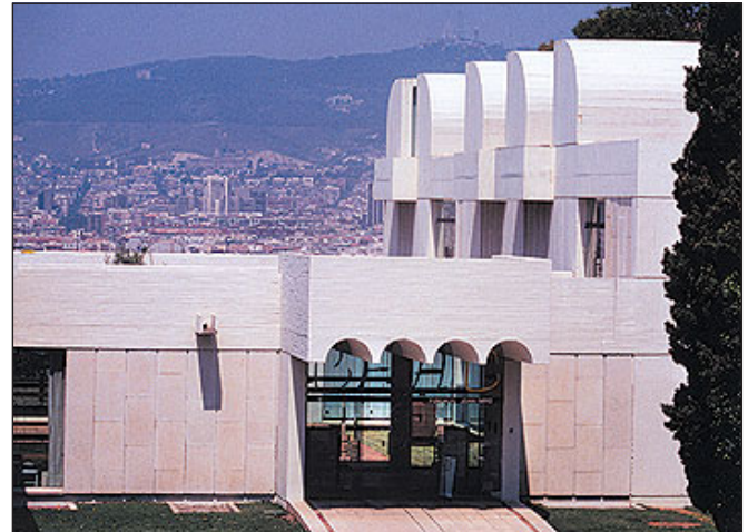
Sert's signature monitors define the museum's profile and direct light deep into the building.
