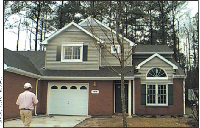
Family housing like this unit at Fort Lee, Va., incorporates sustainable design principles—and typically has a waiting list for residents.
