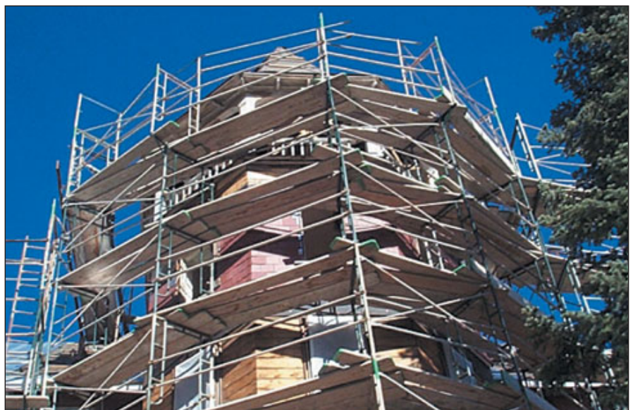
The castle's distinctive brick turrets had to be completely rebuilt.
