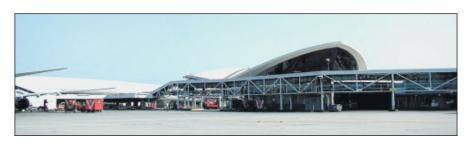
Port Authority's original plan. Most significantly, the agency reworked its roadways into a fairly complex pattern that includes a departure lane that takes cars under the TWA Terminal's umbilical jetways, allowing the umbilicals to be saved. Preservation of the jetways allows for preservation of Saarinen's original parti, which called for entry into the main building and a processional departure down long hallways to a destination—now to be the new terminal.
