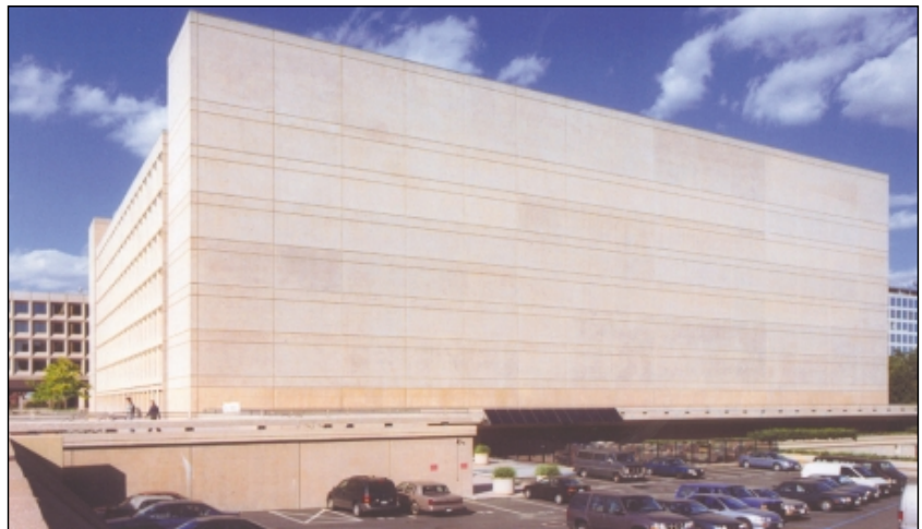
U.S. Department of Energy Forrestal Building (1968) may get a PV-array retrofit.
