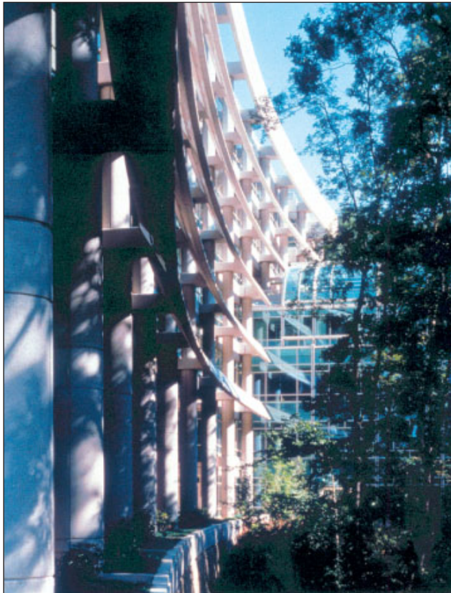
United Parcel Service World Headquarters, Atlanta.
