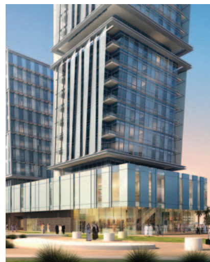
Riyadh, Saudi Arabia, Mixed Use Tower - Solar Shading
