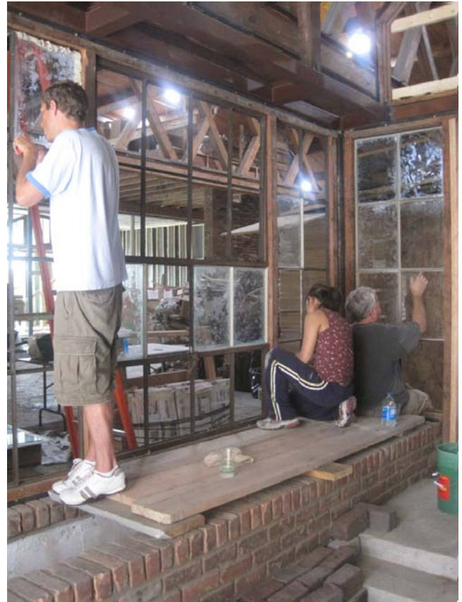
QEA Re-glazing windows at the Green Garage
