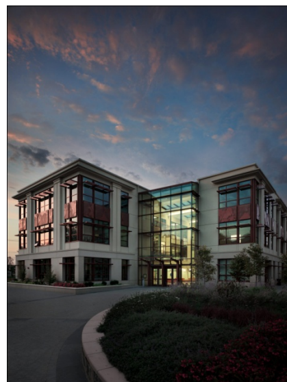
American University School of International Service Tracking: LEED NC Gold
